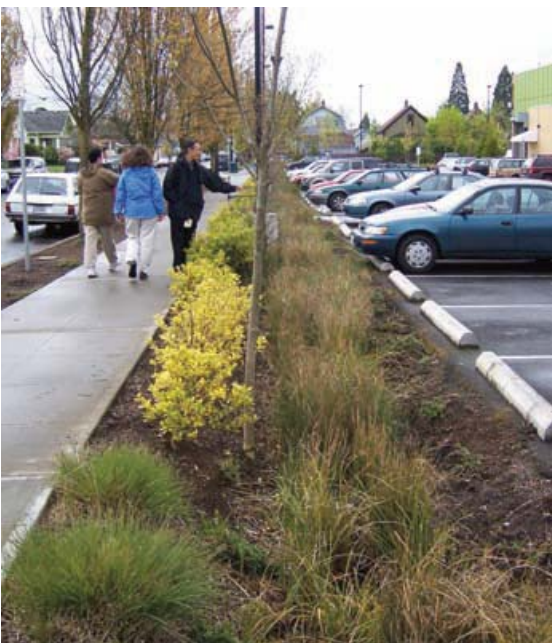
Photo (left): In addition to managing runoff from the parking lot, this bioswale provides an attractive landscaping feature appreciated by pedestrians. Photo (top): High Point received a National Award for Smart Growth Achievement in 2007 from the EPA.
