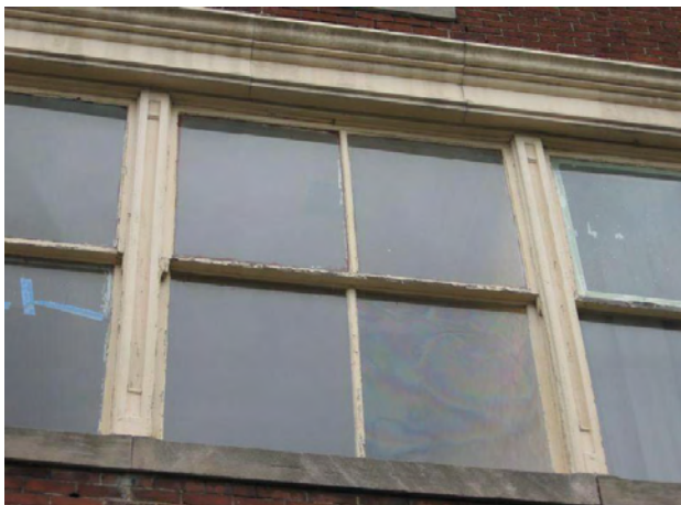
Historic windows like these at 115 North Third Street should be retained and repaired.
