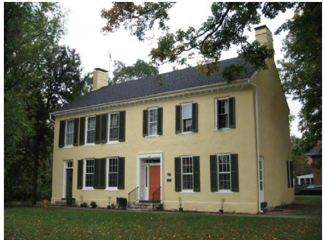
Another Federal house is this one at 103 East Stephen Foster Avenue.
