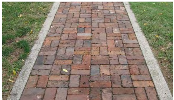
Bricks like those used in the 200 block of West Flaget Avenue are the preferred materials for replacement sidewalks in much of the district.
