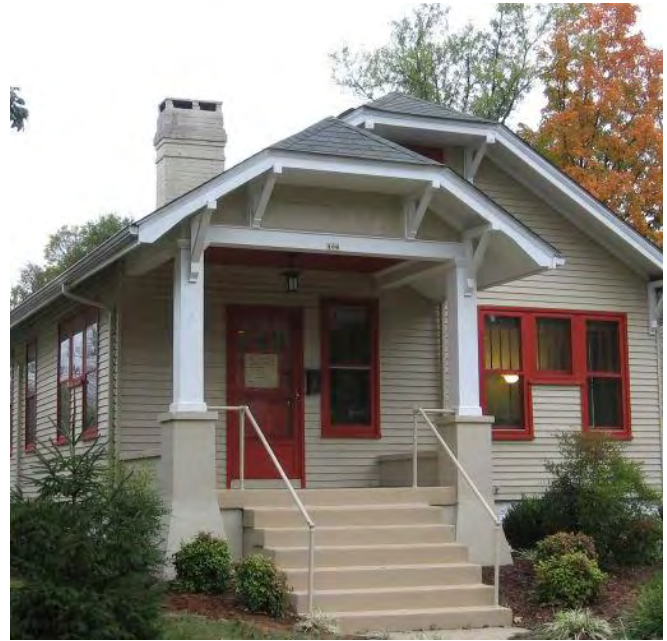
The historically open nature of this porch at 106 East Broadway Avenue should be retained.
