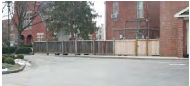
At 101 North Third Street, the fence screens a parking lot and HVAC system from view. (NCPZ Digital Archive)
