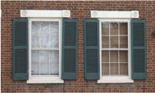
511 North Third Street
