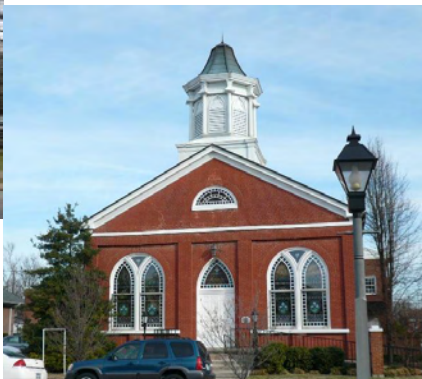
United Methodist Church, 116 East Flaget Avenue (NCPZ Digital Archive)
