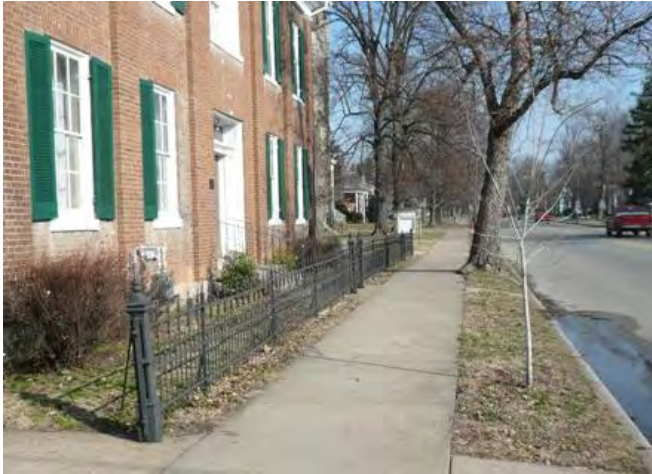
314 North Third Street (NCPZ Digital Archive)
