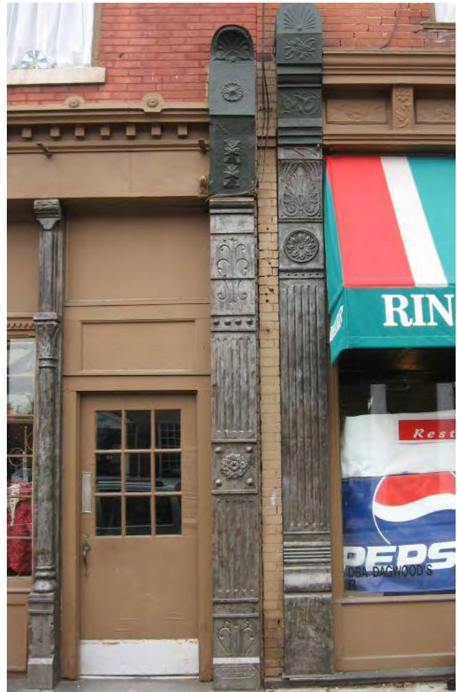
Cast iron architectural features, like pilasters and cornices, decorate commercial buildings like those at 202 and 204 North Third Street.
