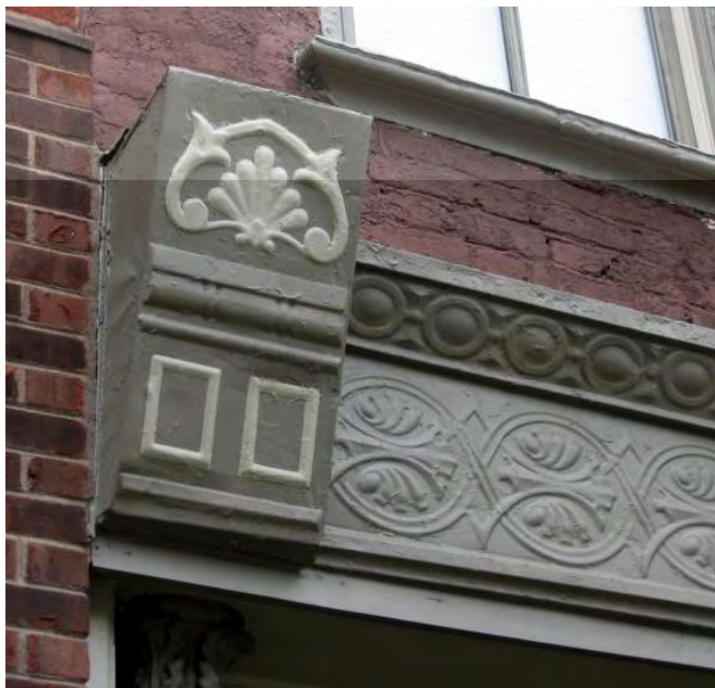
126 North Third Street
