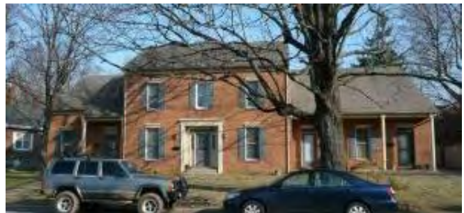
The modern house at 102 West Brashear Avenue followed the historic design and materials precedents set by its neighbors. (NCPZ Digital Archive)
