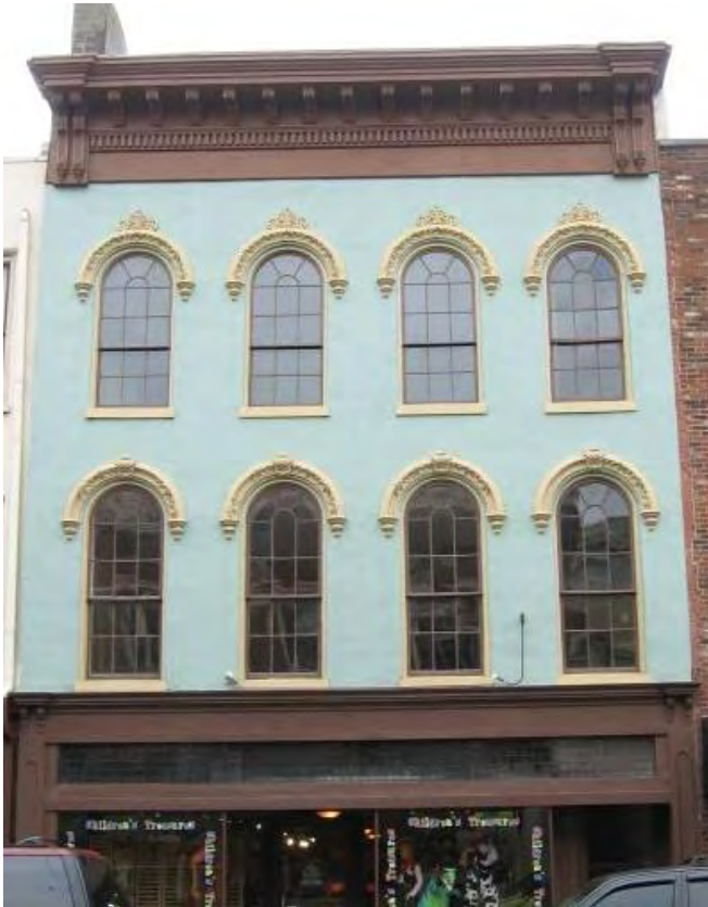
116 North Third Street
