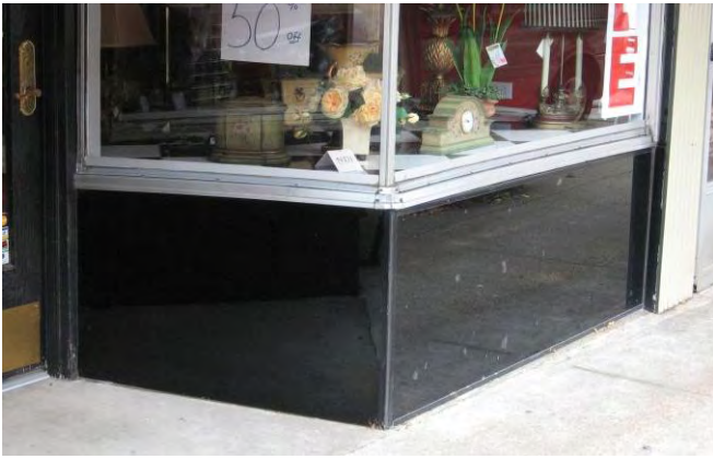
This bulkhead at 125 North Third Street is covered with Carrara glass.
