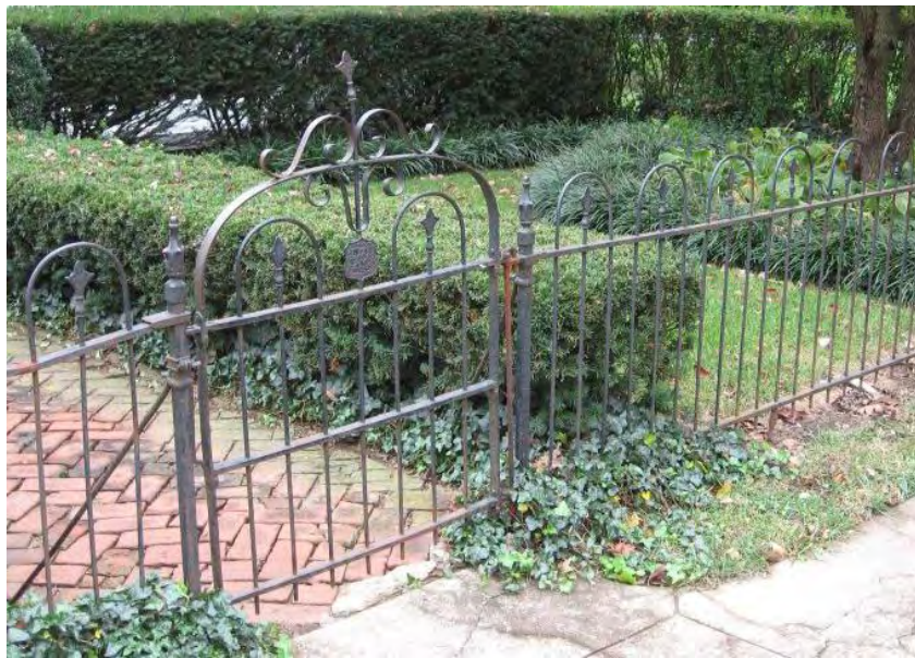
The historic cast iron fence at 207 South Third Street is an appropriate model for new fencing with this pre-1930 house.
