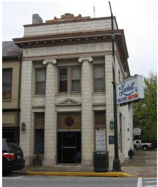
The masonry surfaces of 101 North Third Street should be protected from damaging treatments.
