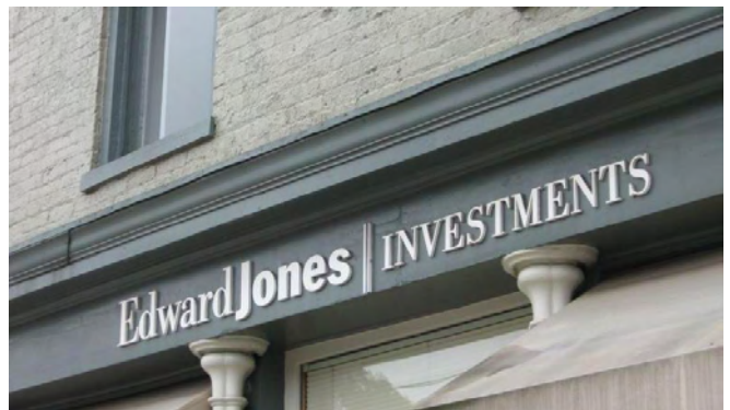
Some storefronts, like the one at 229 North Third Street, have their own cornices and sign panels.
