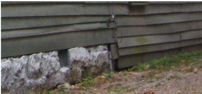
The different foundations at 208 North Fourth Street demonstrate the house's evolution.
