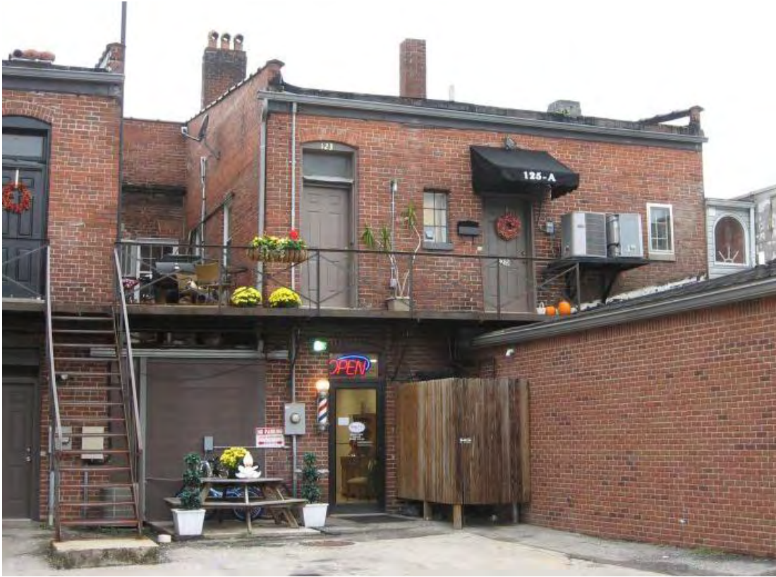
123—125 North Third Street
