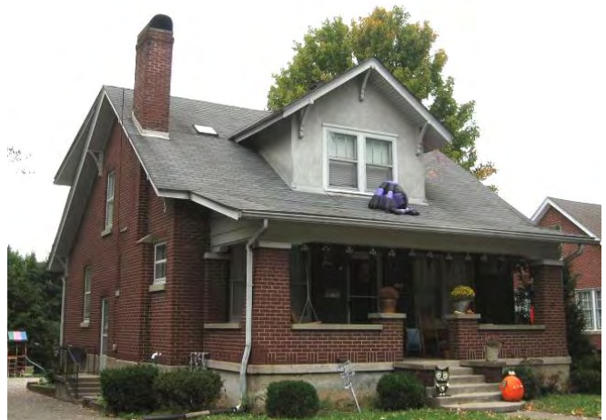
The brick body, concrete trim, and stucco surfaces of the house at 108 South Fifth Street should remain unpainted.
