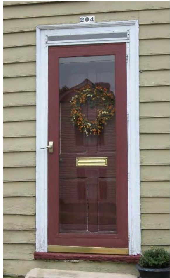
The storm door on 204 West Flaget Avenue uses appropriate materials and design.
