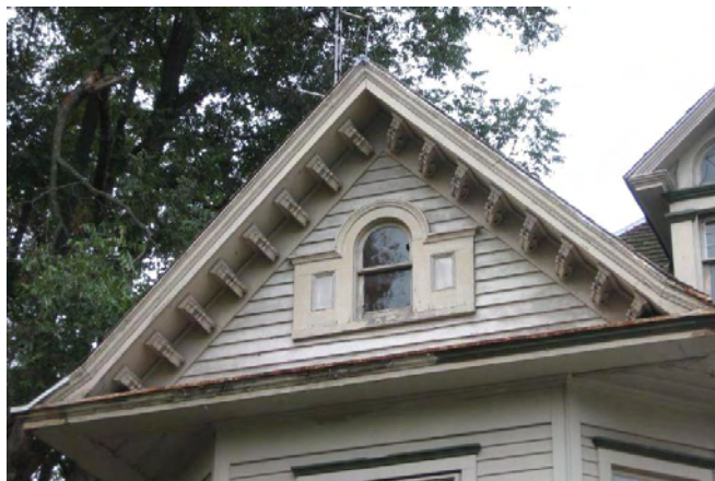
The brackets and window trim provide Italianate and Colonial Revival flourishes to the Queen Anne house at 112 South Third Street and should be retained as important parts of its varied stylistic character.
