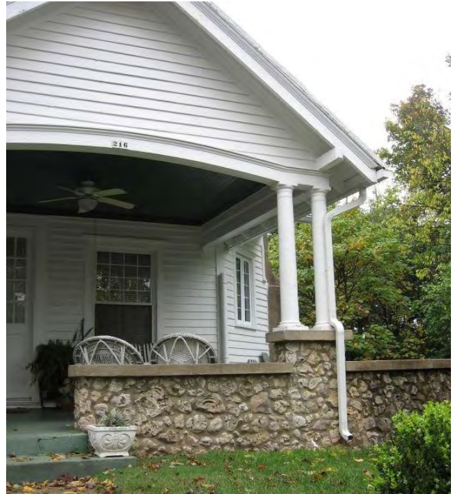
The combination of materials on this porch at 216 East Flaget Avenue includes a cobblestone and concrete railing and paired Tuscan columns.
