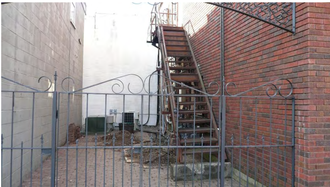
131 North Third Street (NCPZ Digital Archive)
