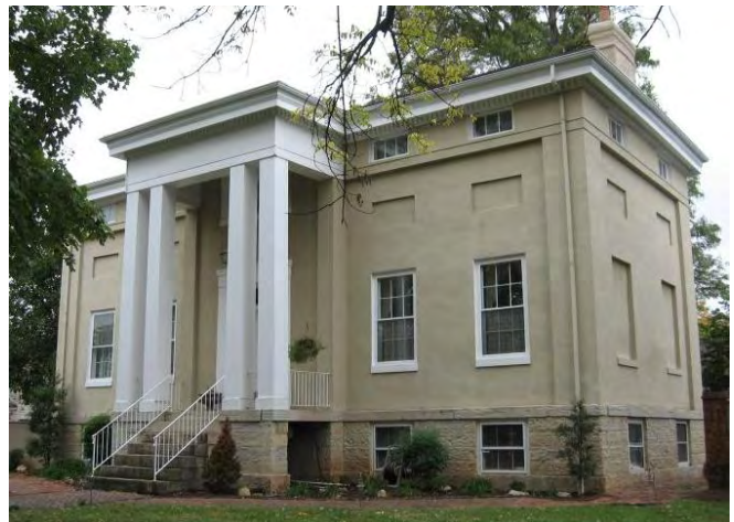
The house at 402 North Third Street has many Greek Revival features, including a low pitched roof, a porch with prominent columns, a cornice line of the roof emphasized with a wide divided band of trim, and a front door surround.
