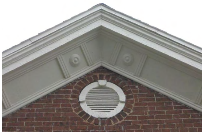
Cornices like this one at 203 South Third Street should be retained.
