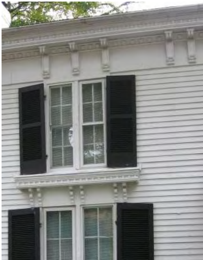
501 North Third Street
