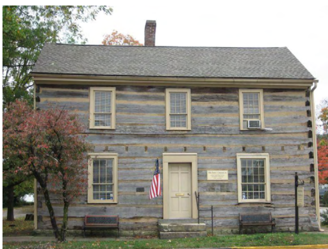
Log houses, such as the Yocum-Hite House at 201 East Stephen Foster Avenue, should retain their unpainted body surfaces.
