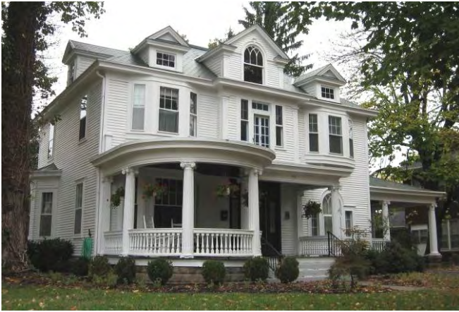
This early Colonial Revival house at 502 North Third Street demonstrates Federal and Georgian influences in its pedimented dormers, arched windows, transom-and-sidelights opening surround, and Ionic capitals. The asymmetry created by its porches was influenced by the Queen Anne style.
