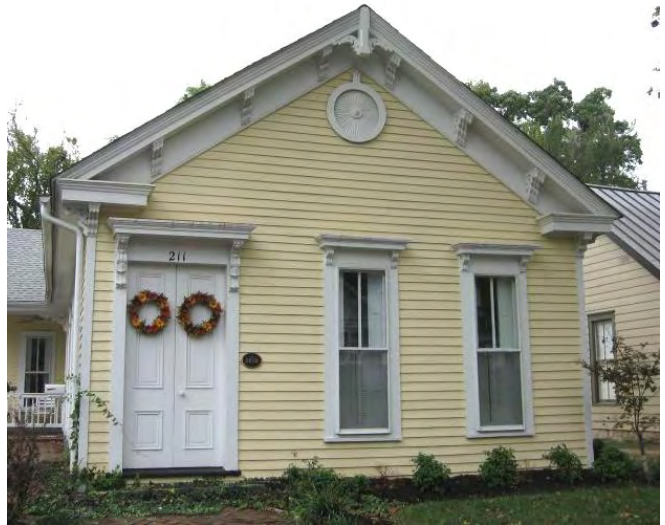
This Italianate house at 211 East Flaget Avenue has overhanging eaves, cornices, brackets, and fascia boards.
