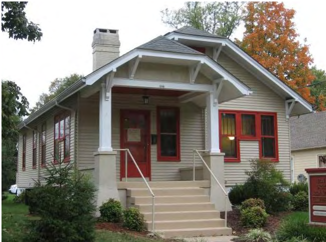
This Bungalow at 106 East Broadway Avenue has roof brackets, multi-light-over-single-light windows, and wood porch posts over flared piers.
