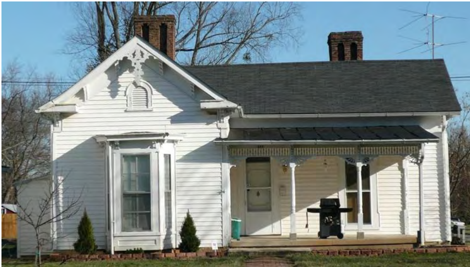
This vernacular gable-front-and-wing house (circa 1885) at 117 South Second Street has Folk Victorian stylistic details such as Steamboat Gothic trim, brackets, and cornice returns. (NCPZ Digital Archive)
