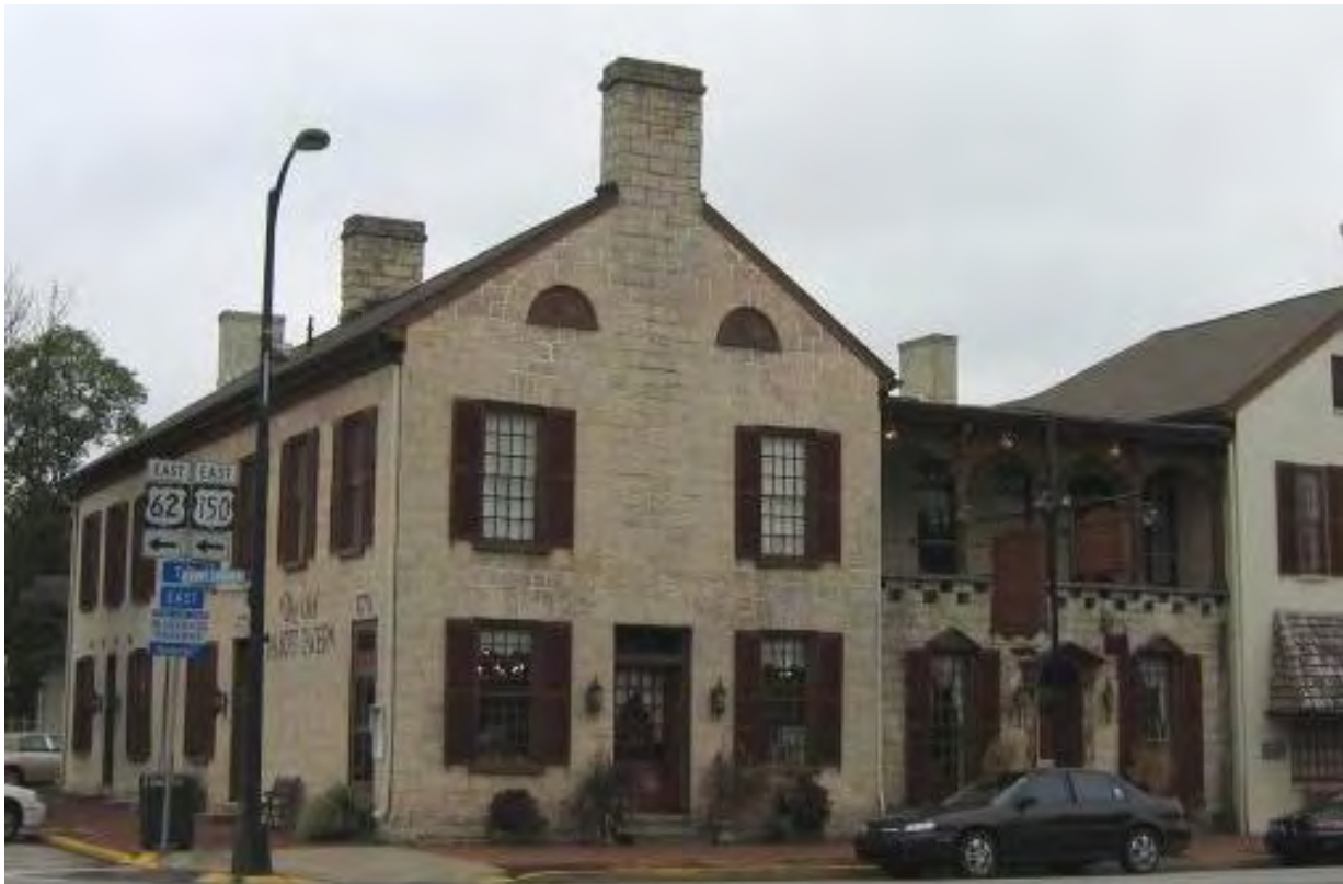
Stone surfaces such as on Talbott Tavern should be left exposed, not painted.
