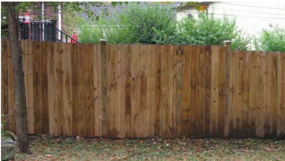
Solid wood fences, like the one at 204 South Third Street, may be used in side and back yards where not visible from the street.
