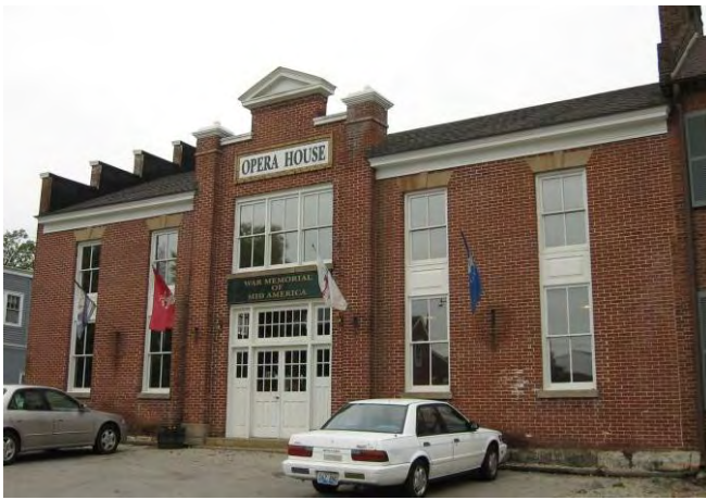
If the brickwork at the Opera House needs to be re-pointed, the original mortar profile should be examined, then replicated.
