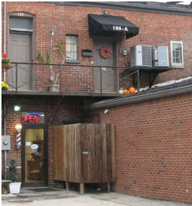
123—125 North Third Street
