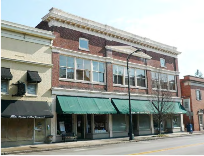
111 North Third Street
