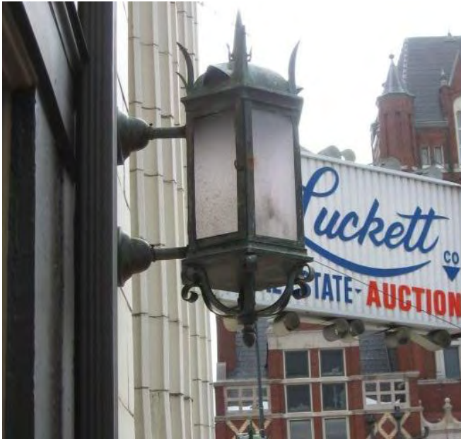
101 North Third Street
