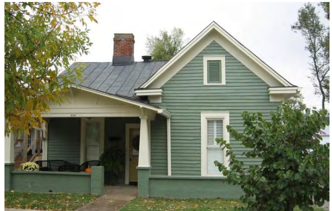
The house at 214 East John Fitch Avenue uses a one-story gable-front and wing plan. Its cornice with returns demonstrates Italianate or Greek Revival influences, and the porch, built in the early 20th century, is Craftsman style.
