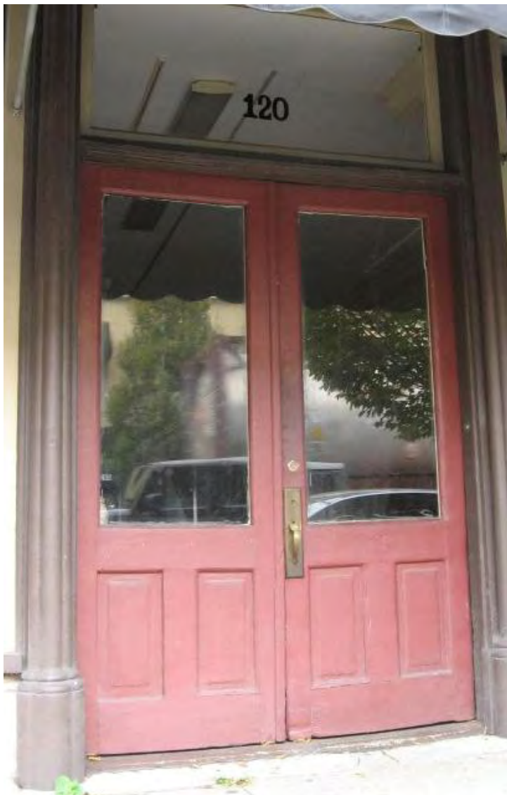
Double doors like 120 North Third Street's were commonly employed for historic storefront entrances.
