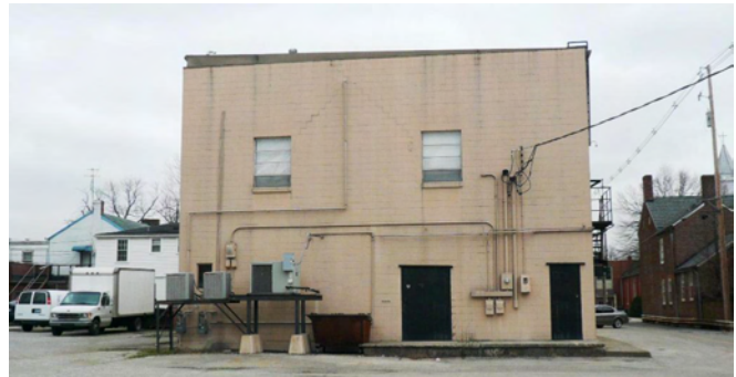
The rear elevations of buildings like this one at 222 North Third Street are appropriate locations for meters and other support elements. (NCPZ Digital Archive)
