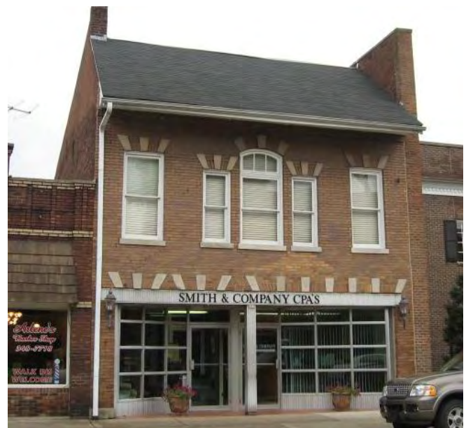
The Old City Hall building at 207 North Third Street is an example of the Colonial Revival style and features a side-gabled roof, symmetry, and three-part window grouping.
