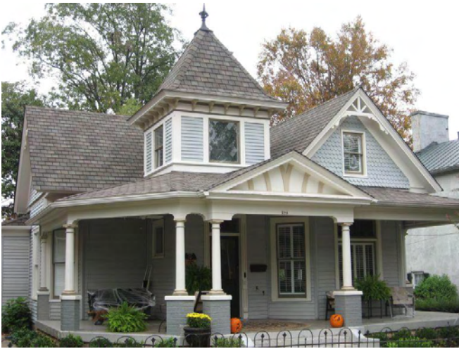
The house at 204 South Third Street has many Queen Anne elements including a tower, decorated gable field, porch, and various heights and projections of building bays.
