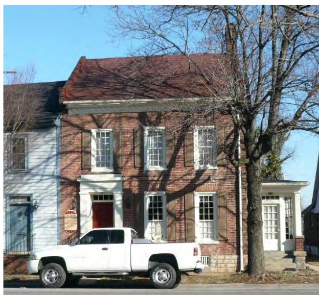
The brick body of the house at 116 East Stephen Foster Avenue should remain unpainted. (NCPZ Digital Archive)
