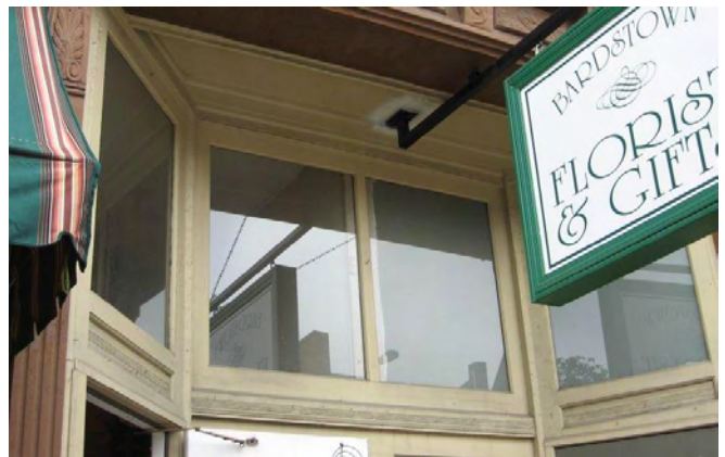
206 North Third Street's transom is recessed and has multi-pane plate-glass installed.
