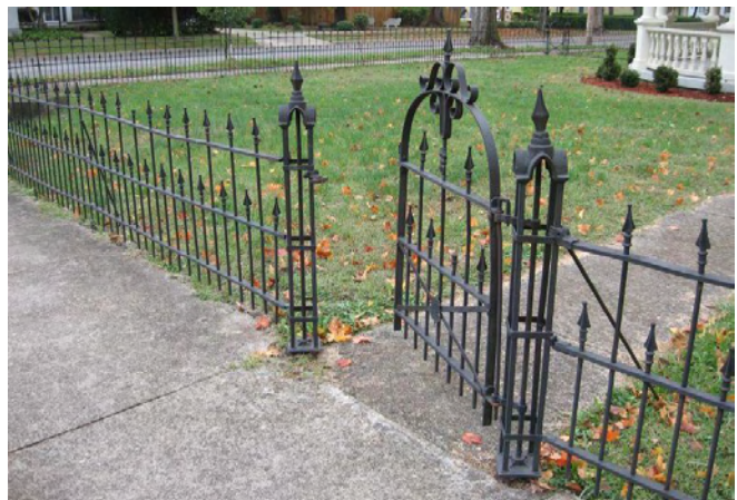
Historic cast iron fences like this one at 114 South Third Street should be retained and repaired.
