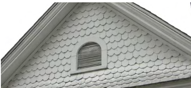
Decorative siding materials like the hexagonal wooden shingles on 202 West Flaget Avenue should be retained and repaired.
