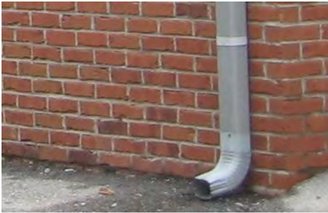
123—125 North Third Street
