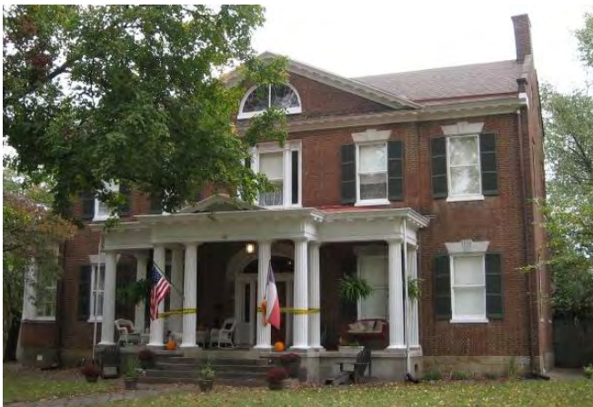
Bardstown architect and builder Osso Stanley added this Greek Revival porch, with pediment, block modillions, and Doric columns, to Shadowlawn, a Federal style home built in 1825 by noted architect John Rogers.
