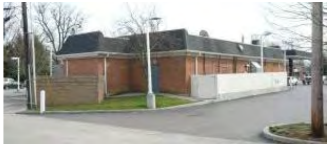
This fence at 122 East Stephen Foster Avenue screens a dumpster and utilities equipment. (NCPZ Digital Archive)
