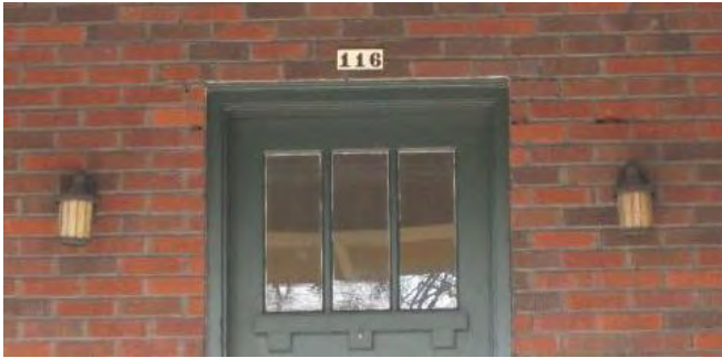
116 North Third Street
