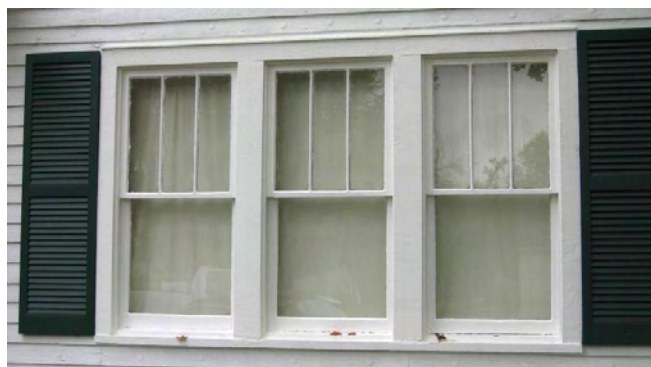
Historic windows like these vertical sash Craftsman designs at 216 East John Fitch Avenue should be retained and repaired.
