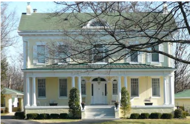
The Dant House (circa 1910), at 211 South Third Street, is an example of a larger Colonial Revival house with its symmetry, accented entryway, double-hung multi-paned windows, and side-gabled form. (NCPZ Digital Archive)
