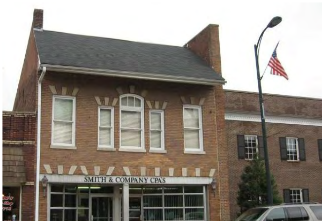
The gable roof on the Old City Hall at 207 North Third Street contributes to its architectural style.
