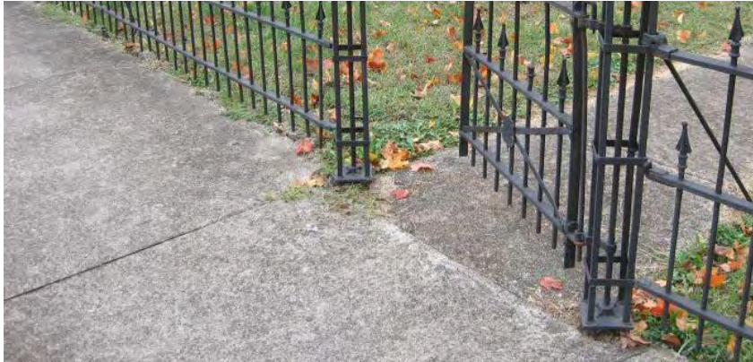
114 South Third Street
