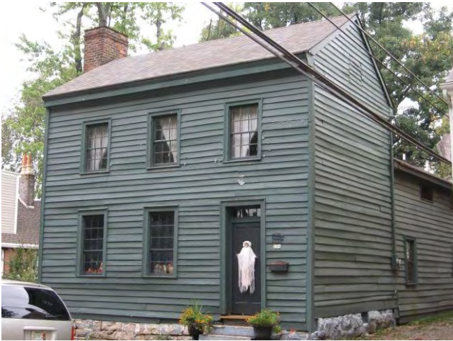
The Rizer House at 208 North Fourth Street, constructed circa 1820, is two stories, proportionally balanced, and has a plain appearance. This house has a frame rear wing and weatherboard siding, with infill in the ell.
