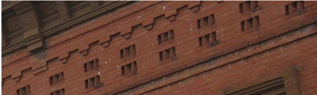
The brick corbelling in the 200 block of North Third Street helps to define historic character.
