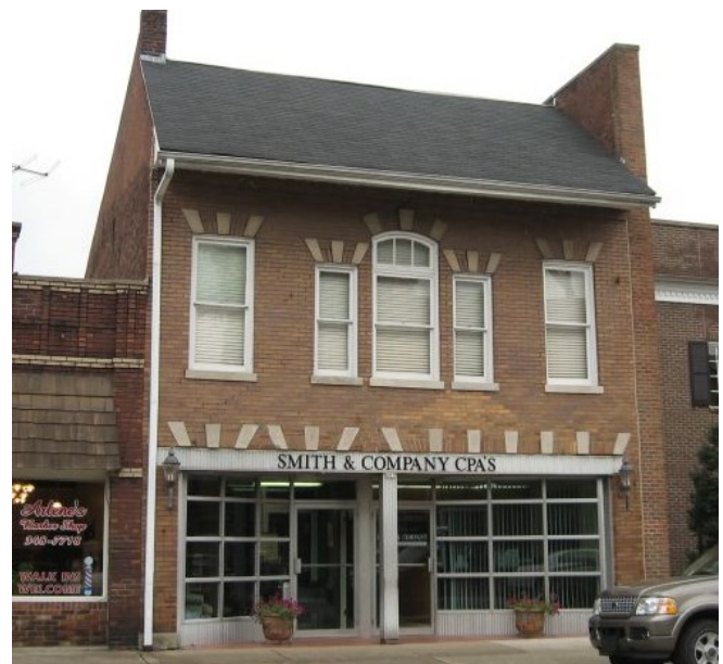
The Old City Hall building at 207 North Third Street is an example of the Colonial Revival style and features a side-gabled roof, symmetry, and three-part window grouping.
