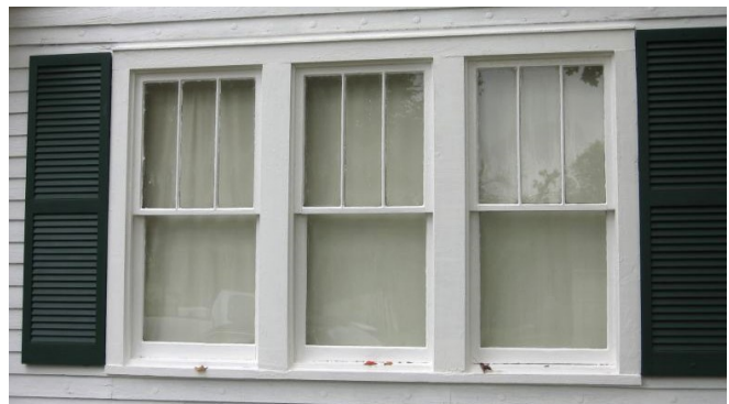
Historic windows like these vertical sash Craftsman designs at 216 East John Fitch Avenue should be retained and repaired.
