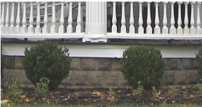
The carefully textured finish on the foundation stones at 502 North Third Street shows the house's turn of the century construction.
