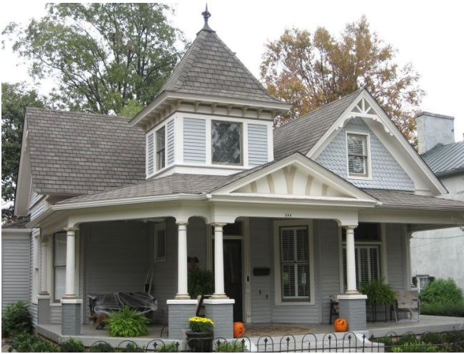
The house at 204 South Third Street has many Queen Anne elements including a tower, decorated gable field, porch, and various heights and projections of building bays.
