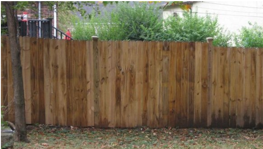
Solid wood fences, like the one at 204 South Third Street, may be used in side and back yards where not visible from the street.
