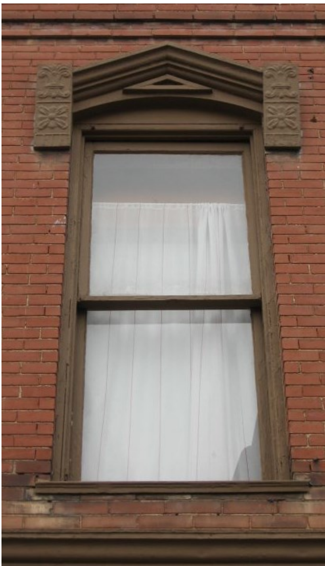
Retaining the painted finish of the wooden window sash at 204 North Third Street contributes to historical character and building maintenance.
