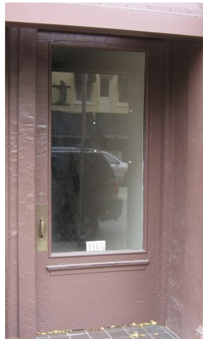
Single doors like the one at 116 North Third Street were often used for secondary commercial entrances.
