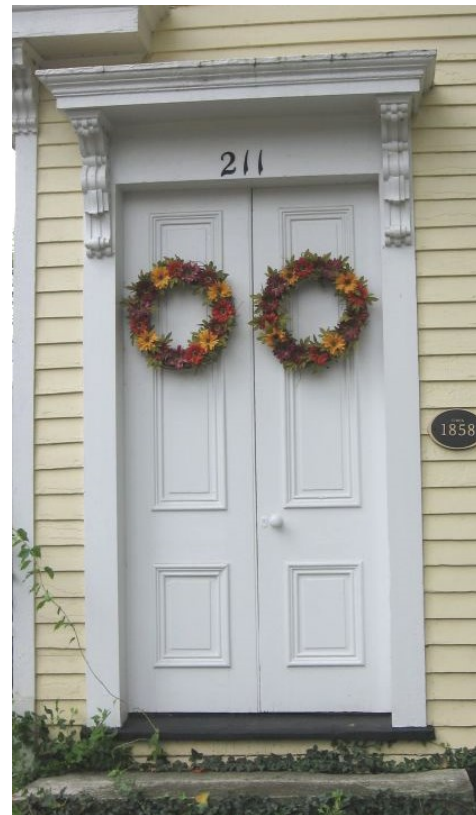
The paired paneled wooden doors at 211 East Flaget Avenue have a Classical-inspired surround.
