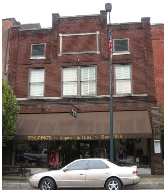
The contrast between concrete and brick is the main decorative feature of the building at 122 North Third Street.
