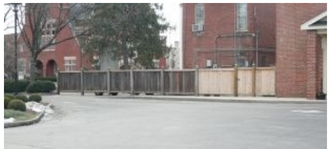
At 101 North Third Street, the fence screens a parking lot and HVAC system from view. (NCPZ Digital Archive)
