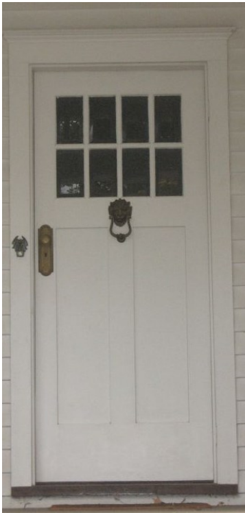
Historic doors like the one at 210 East Flaget Avenue help define the historic character of buildings and neighborhoods.
