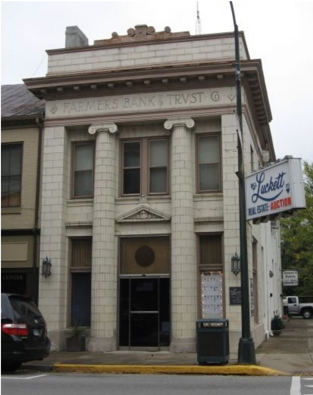
This bank building at 101 North Third Street has a symmetrical façade, pilasters extending the height of the building, Ionic capitals, and a pediment over the entrance—all indicators of the Neoclassical style.
