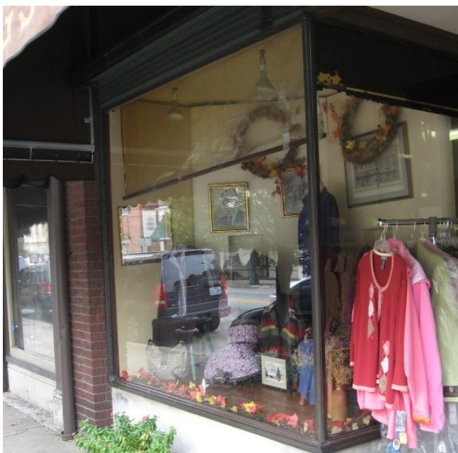
Original or historic display windows such as those at 122 North Third Street should be preserved and maintained.
