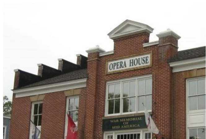
Roofline details contribute to the character of the Opera House.
