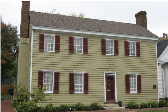
The Jacob Rizer House at 204 West Flaget Avenue was built circa 1802 and displays the center-hall plan with paired end chimneys.
