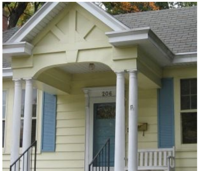
Lighting placement on the porch roof at 206 East Flaget Avenue is appropriate.
