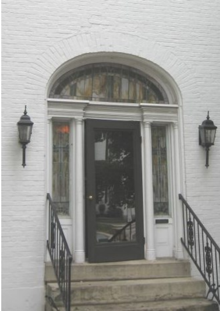
The entrance at 212 East Stephen Foster Avenue contributes to the building's Federal style.
