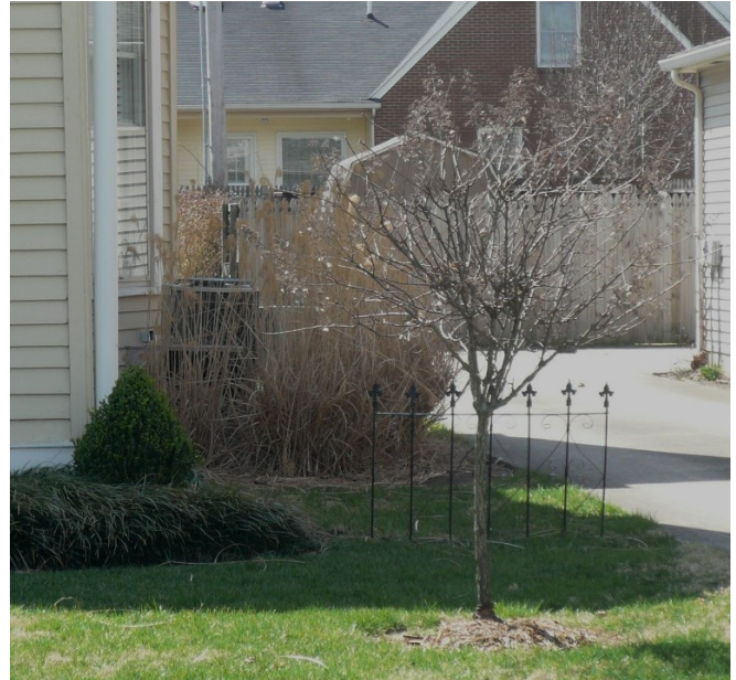
Plants and landscape elements help shield the air-conditioning unit at 213 West Broadway Avenue from view.
