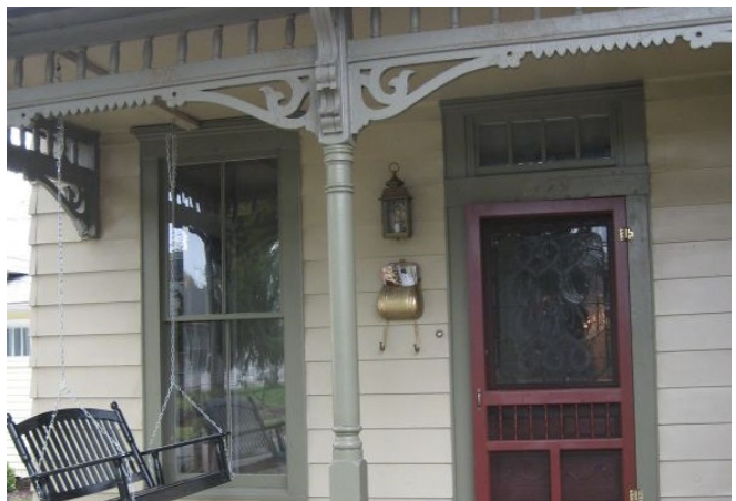
The placement of the lighting fixture alongside the entryway at 209 East Flaget Avenue is appropriate.
