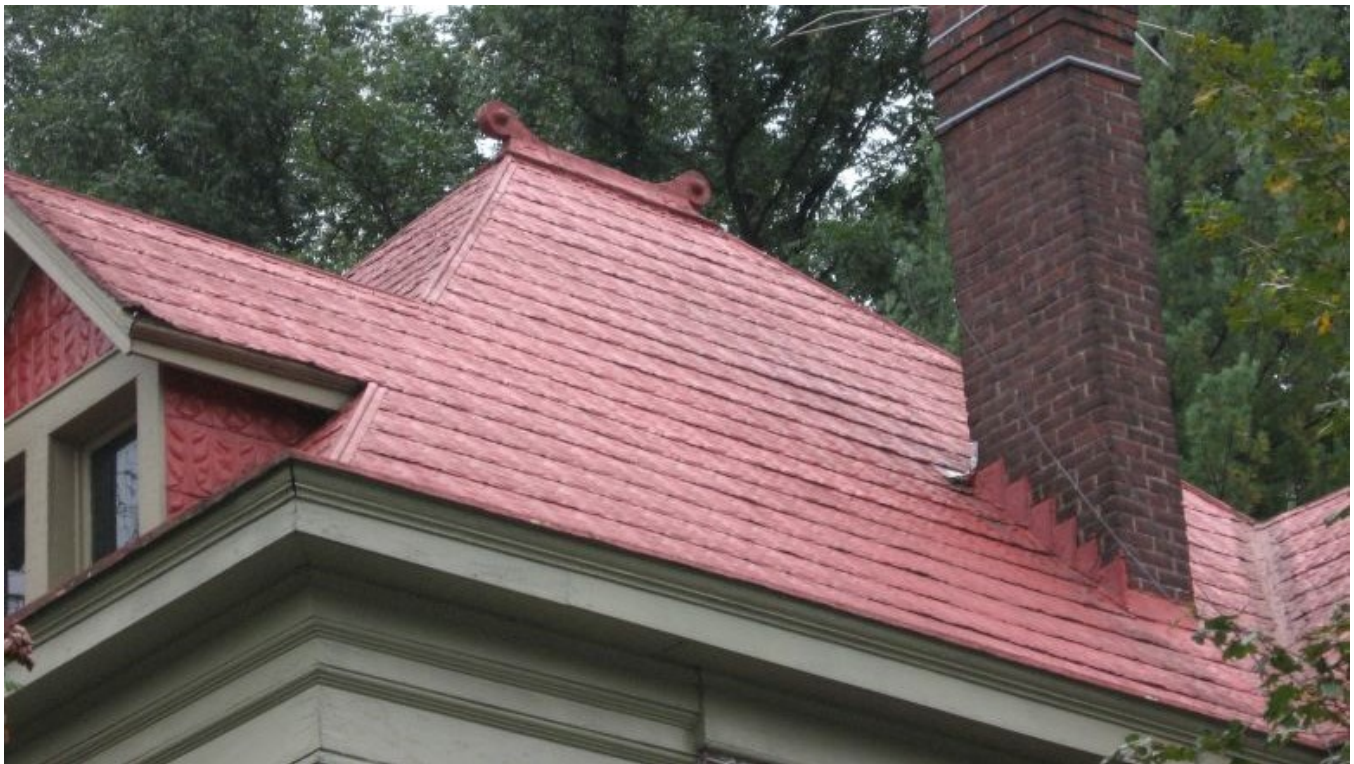
Creasting and pressed-metal shingles add to the historic character of the house at 117 West Broadway Avenue.
