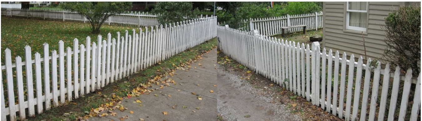
The design, materials, and color of the wood picket fences at 113 East Brashear Avenue (left) and 317 Raspberry Alley (right) are appropriate.
