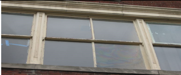
Historic windows like these at 115 North Third Street should be retained and repaired.
