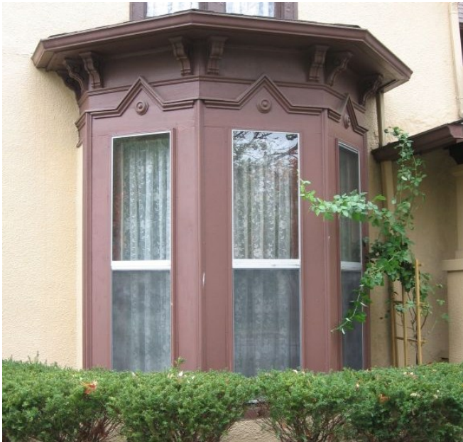
208 South Third Street
