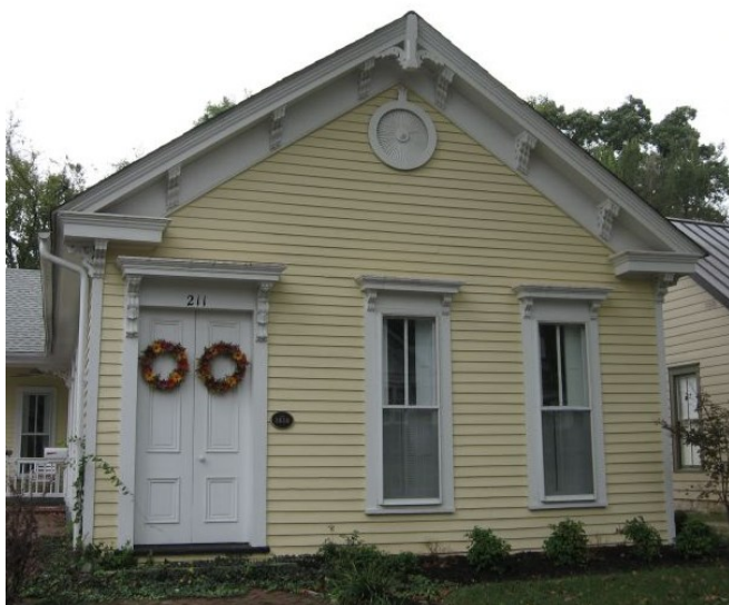
Brackets, gable returns, and window and door cornices all help define the mid 19th century Italianate style of the house at 211 East Flaget Avenue and must be retained to protect its integrity.
