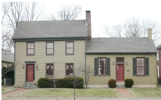
The Federal house at 110 East Broadway Avenue has a subdued color scheme and retains a painted finish on traditionally painted wooden elements. (NCPZ Digital Archive)
