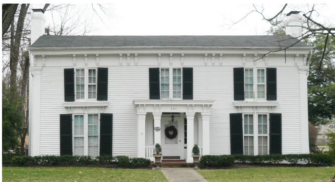
The house at 501 North Third Street is a good example of Italianate residential architecture. (NCPZ Digital Archive)
