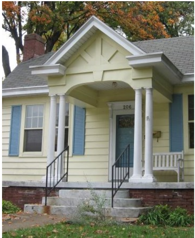
The paired columns, simple Tuscan capitals, cornice returns, and size of the porch on 206 East Flaget Avenue are Colonial Revival elements.
