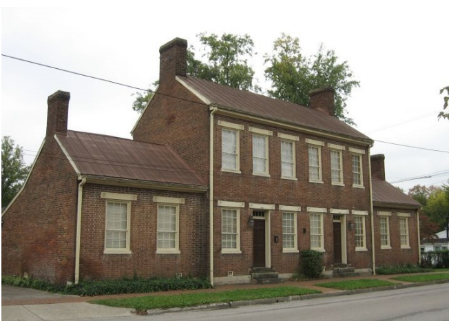
This duplex at 205 and 207 West Flaget Avenue combines an urban form with the Federal style.
