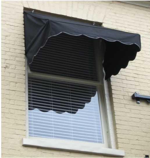
This replacement window at 117 and 119 North Third Street is appropriate.
