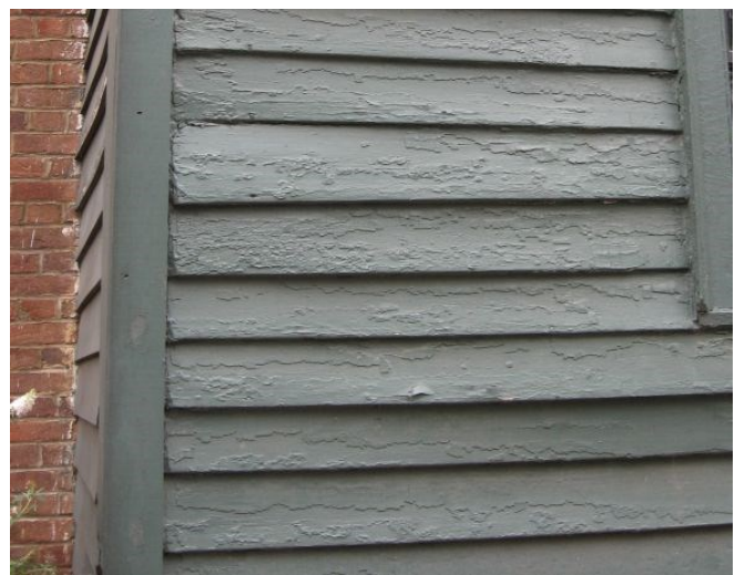
This weatherboard siding at 208 North Fourth Street is almost 200 years old; its appearance adds greatly to the historic character of the property.
