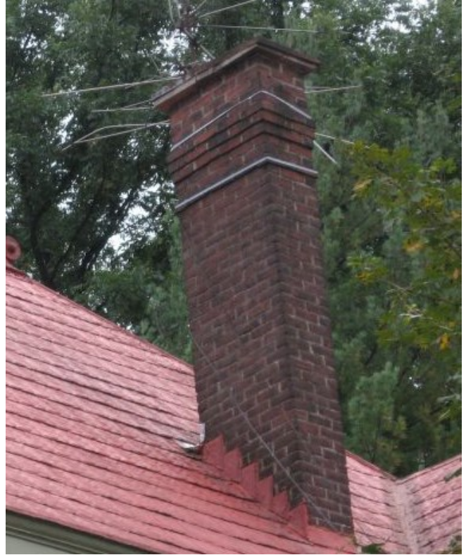
The chimney on the house at 117 West Broadway Avenue is an important feature and should be retained.
