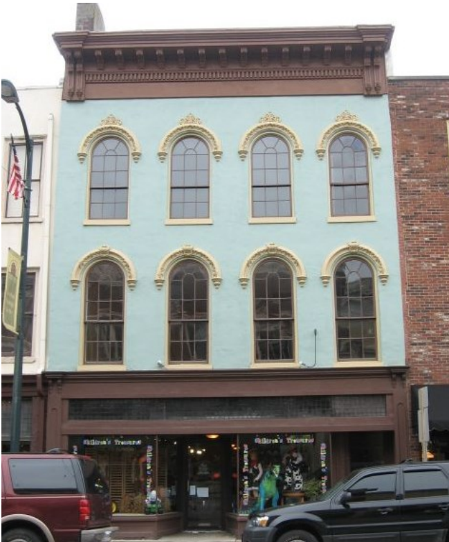
This Italianate style commercial building at 116 North Third Street has arched windows and hoods and a bracketed cornice.
