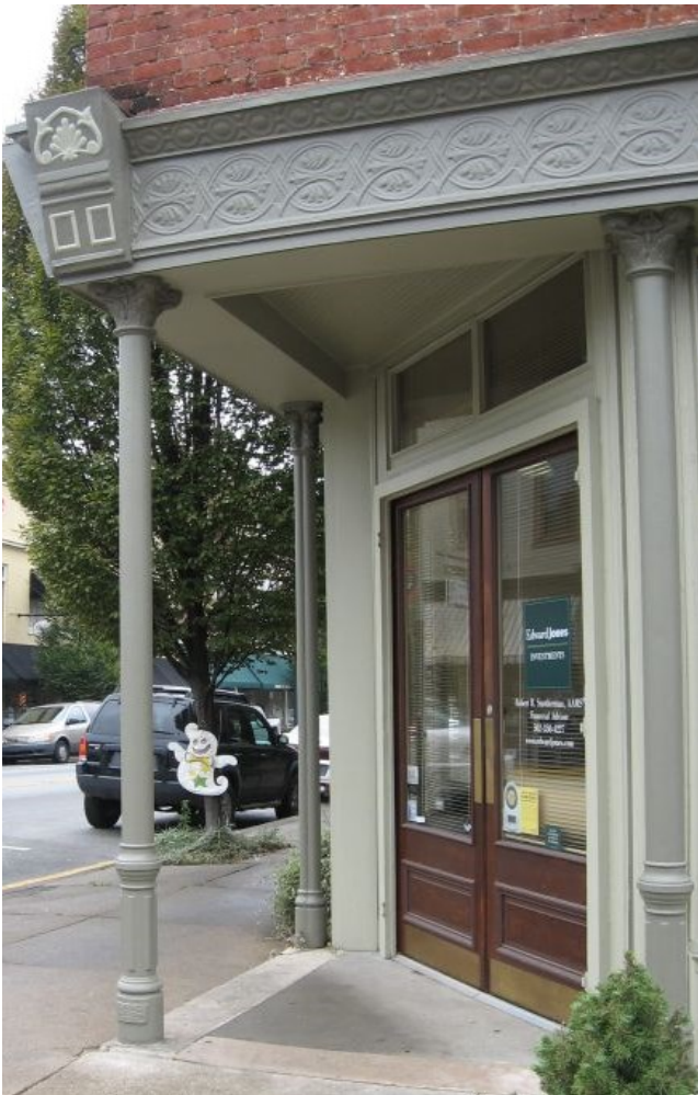
Maintain the painted surface of features like the cast iron columns and pilasters at 130 North Third Street.
