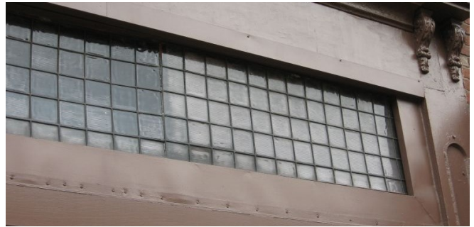
The building at 116 North Third Street has a Luxfer glass transom.
