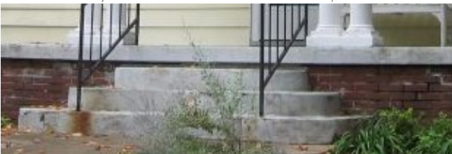
The wooden steps at the upper left, brick steps at the upper right, and concrete steps at 206 East Flaget Avenue all appropriately used materials that matched their porch's materials.
