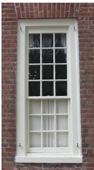
The replacement window at 116 East Stephen Foster Avenue helps to retain the house's historic appearance.
