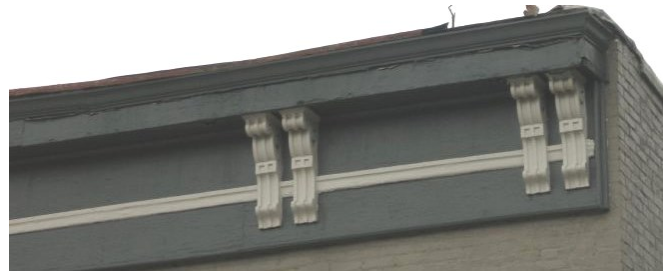
This cornice, at 229 North Third Street, should be retained.
