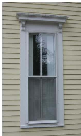
The storm window on 211 East Flaget Avenue is appropriate.
