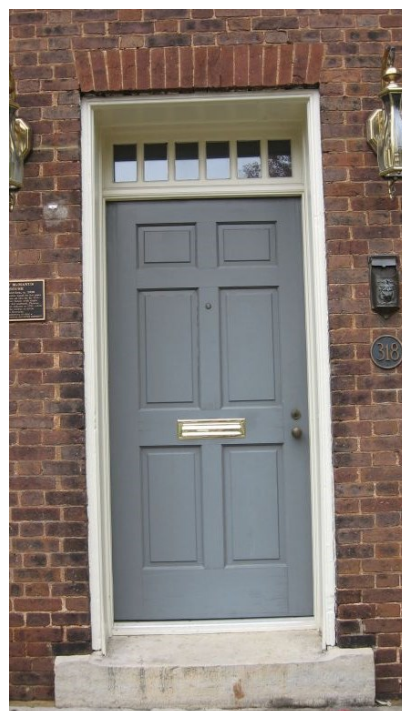
The replacement door on 318 North Second Street used appropriate design and materials.
