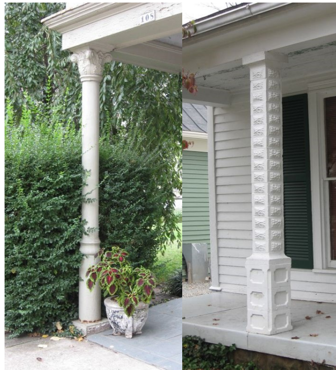
The column at 108 South Third Street and the distinctive post at 216 East John Fitch Avenue are character-defining elements.
