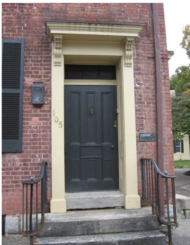
The entrance elements of the McLean House at 105 East Stephen Foster Avenue contribute to its historic character.
