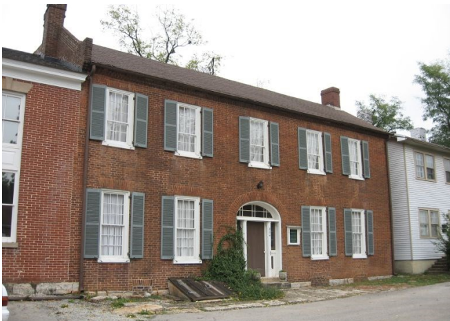
The James Wright House at 204 East Broadway Avenue is a good example of a Federal row house. The sidelights and door surround indicate a transition from Federal to Greek Revival architecture.
