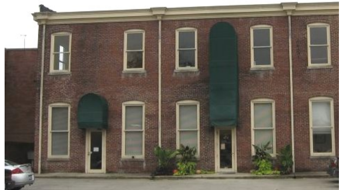
Placement of these gutters and downspouts, on the rear of the building at 111 North Third Street, is appropriate.
