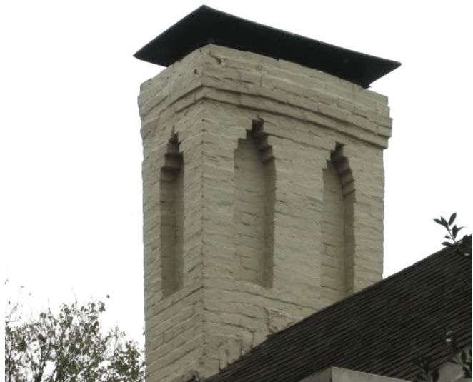
The decorative appearance of chimneys like that at 205 South Third Street should be preserved through repair or replacement.
