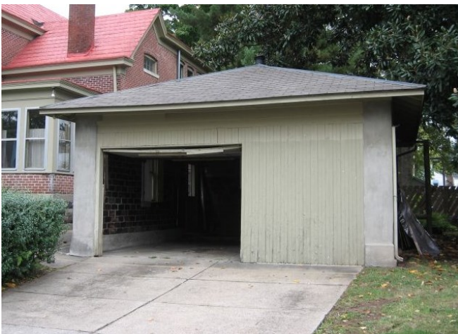
Original garages should be preserved and maintained such as this one at 117 West Broadway Avenue.
