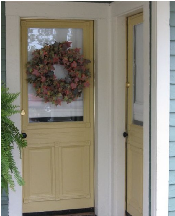
Single-light glass-and-wood doors like these at 204 East John Fitch Avenue were widely used at the turn of the 20th century.
